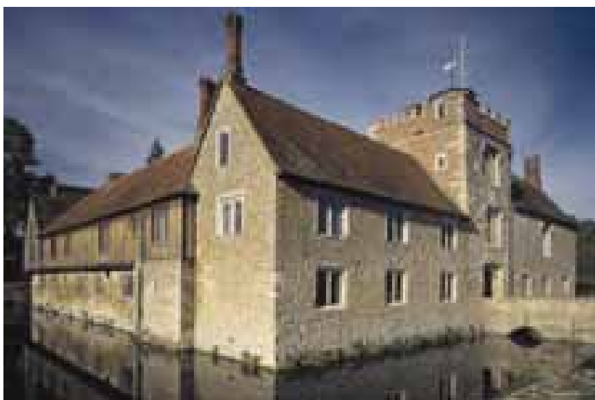
Grants totalling £298,000 were made to the National Trust between 1982 and 2002. Conservation work at Ightham Mote was funded by an award in 2002
