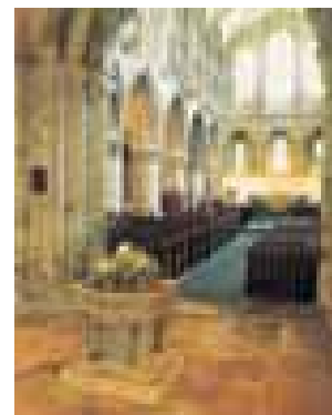
A grant of £4,000 was made in 2004 for repair work at St Mary de Havra, New Shoreham in Sussex
