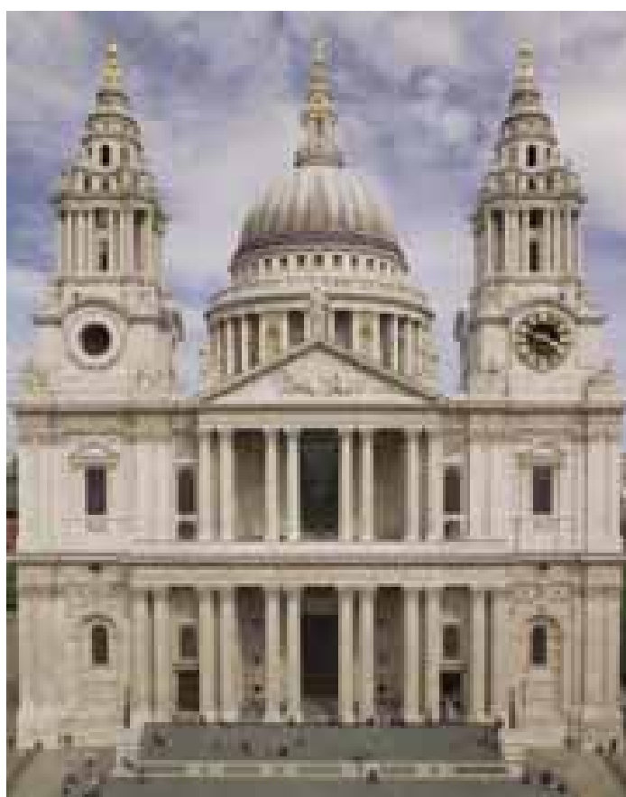
Grant totalling £305,000 were made for repair work at St Paul's Cathedral in 1971, 1994 and 2001 © Sampson Lloyd
